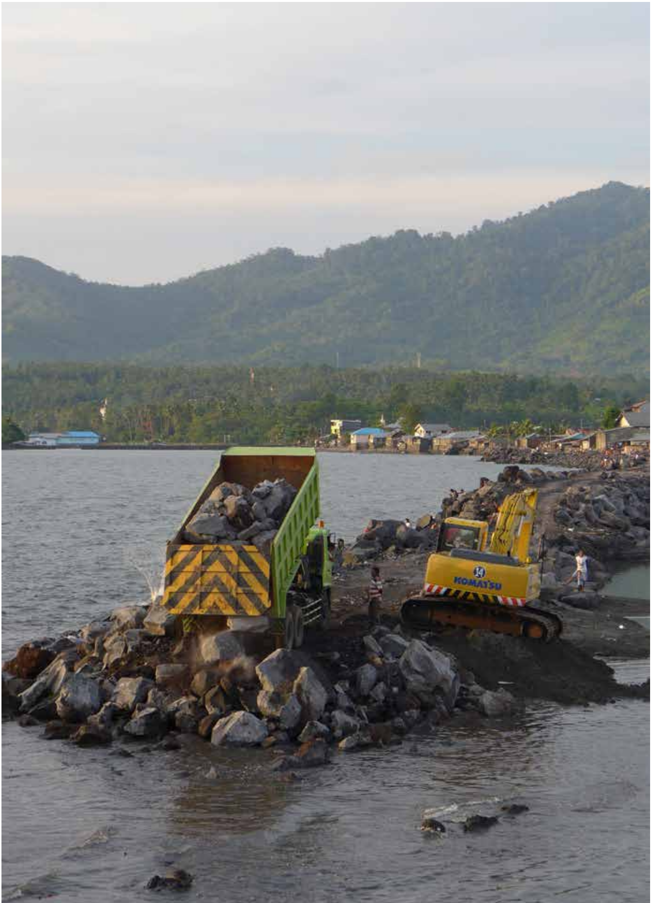
Figure 20: The city government and private sector have focused planning efforts to reshape the coastline and provide improved mobility and opportunities for commercial development. This coastal reclamation has significant impacts on the surrounding fragile ecosystem and also complicates drainage.
