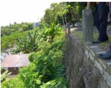
Retaining walls to prevent landslides
